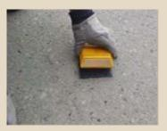
Step 4 Immediately press devise on softened pad and allow cooling, to achieve maximum adhesion, requires only a few minutes
