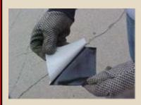
Step 1 Contact Surface must be completely clean, dry and free of foreign and loose material. Pre heat the ground where the adhesive will be placed
