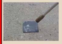
Step 3 Heat the top of the Pad using a standard torch until pad is liquified and the clear plastic is flashed off
