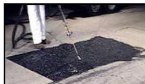
Flood with Concrete Welder.
