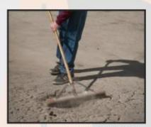
To begin, use a wire brush and compressor to sweep and blow the dirt out of the hole.
