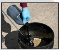
Shake "B" bottle for 30 seconds. Pour into bucket. Mix for 2 minutes.
