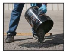
Flow material into damaged area to just-blow grade.
