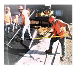
LUTE BARS COME IN 5 SIZES 24"-30"-36"-42"-48"HANDLES AVAILABLE IN 4 LENGTHS  $6' X 1 \frac{1}{2}"$  DIAMETER  $7' X 1 \frac{1}{2}"$  DIAMETER  $8'4" X 1 \frac{1}{2}"$  DIAMETER  $6'9" X 1 \frac{1}{4}"$  DIAMETER FIBERGLASS HANDLES  $8'4" X 1 \frac{1}{4}"$  DIAMETER Fiberglass Handle Tested to a Conductivity Breakdown Point of 58.9 kilovolts
