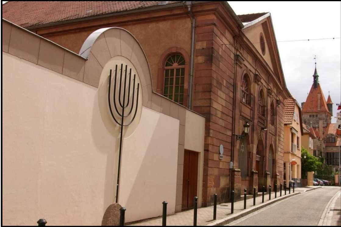
The Synagogue in Haguenau. Constructed in 1820.
