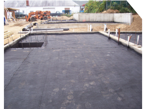
UltraShield™ G-800 is a needle-punched, non-woven geotextile with superior tensile strength and puncture resistance.
