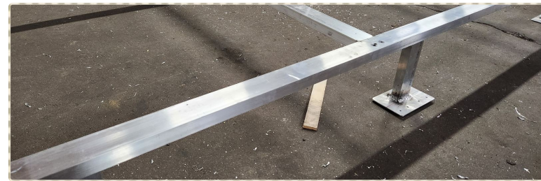
The custom frame, welded from scratch
