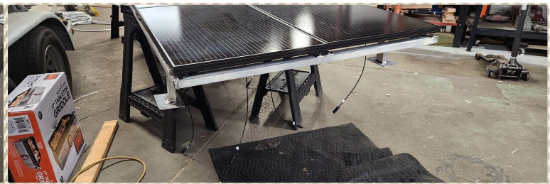
Panels laid out and wired
