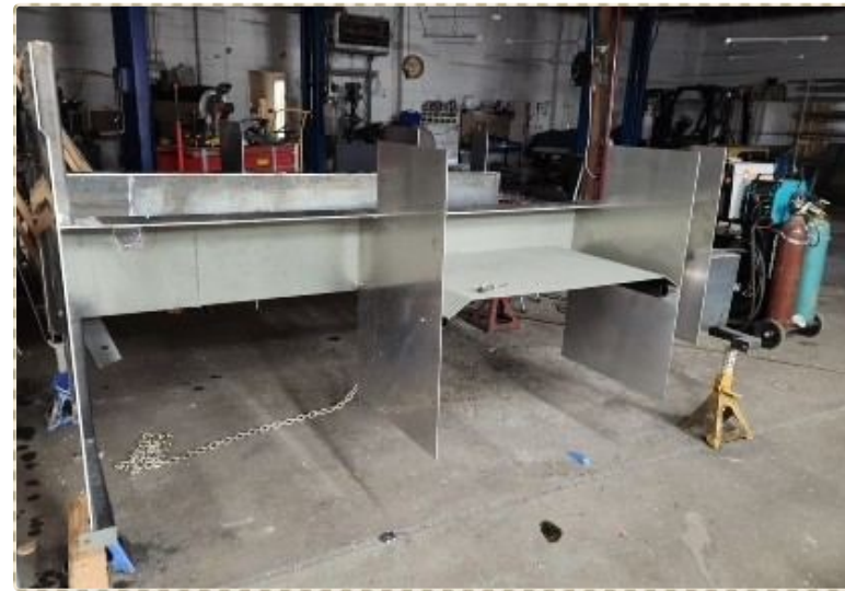
The beginning of the aluminum cabinet structure
