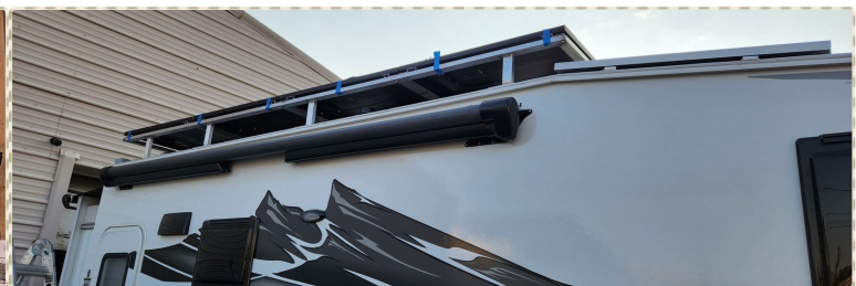
Installed and routed around the roof obstacles
