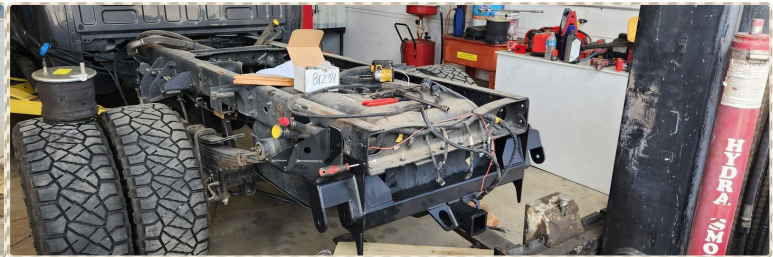
Prepping the frame rails, Kelderman cross member going in
