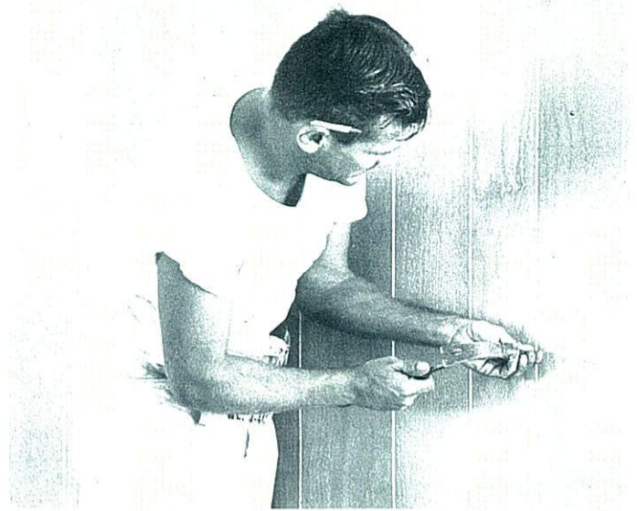
PANELED WALL —A wall is finished in selected wood paneling. Nails are placed and skillfully covered so no nailholes show in finished wall surface.
