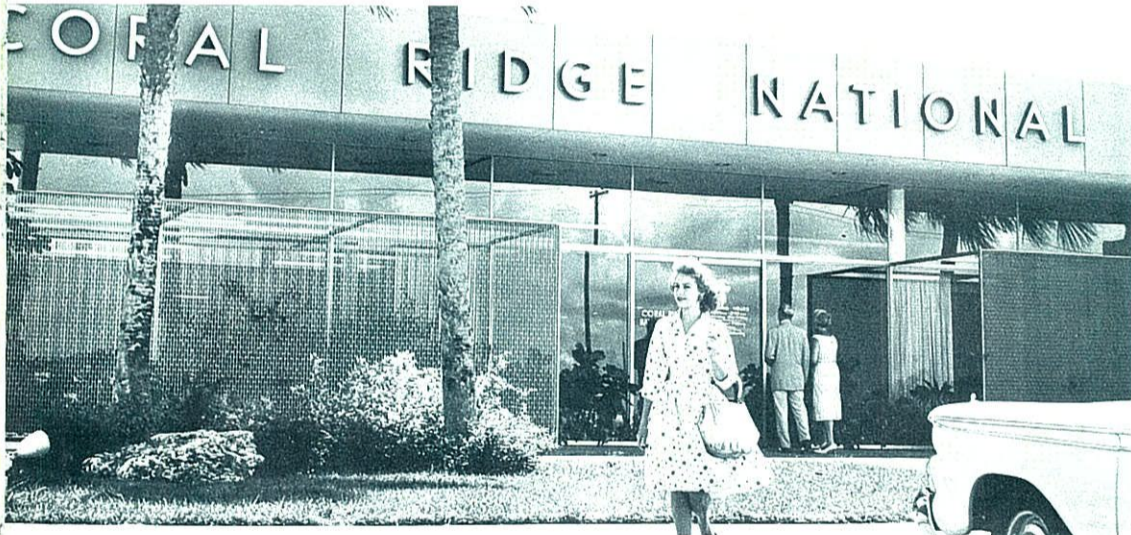
COMMERCIAL BANKS are not permitted to have branches under Florida law. Savings and Loan institutions are. Banks and savings offices are strategically situated throughout Fort Lauderdale - Pompano Beach area. Airy and spacious, with wide
