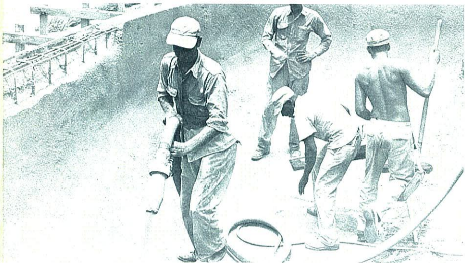
BUILDING A POOL —Concrete is sprayed from guns under high pressure onto swimming pool's steel frame by guniting process. Special gunite process costs the builder more, but produces a stronger, finer pool.
