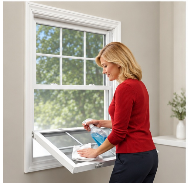
03 Clean the supported lower sash.
