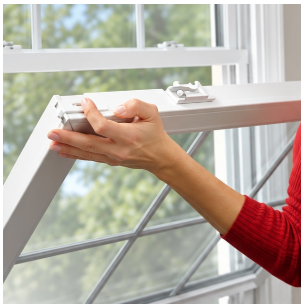
01 Release both tilt latches.
