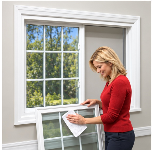
03 Support the removed sash on a safe surface.
