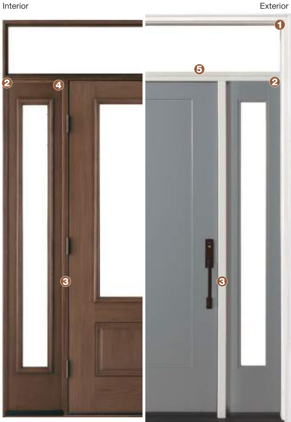
1 Brickmould 2 Jamb 3 Mullions 4 Cove Mould 5 Transom Sill
