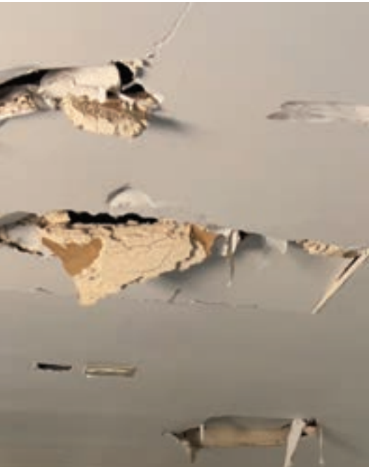
The WaveRunner® had risen up so rapidly and high with a force and speed that must have been great. Not only was it completely destroyed, but much of the garage ceiling was, too. The WaveRunner® did not matter; the risk of structural damage did.
