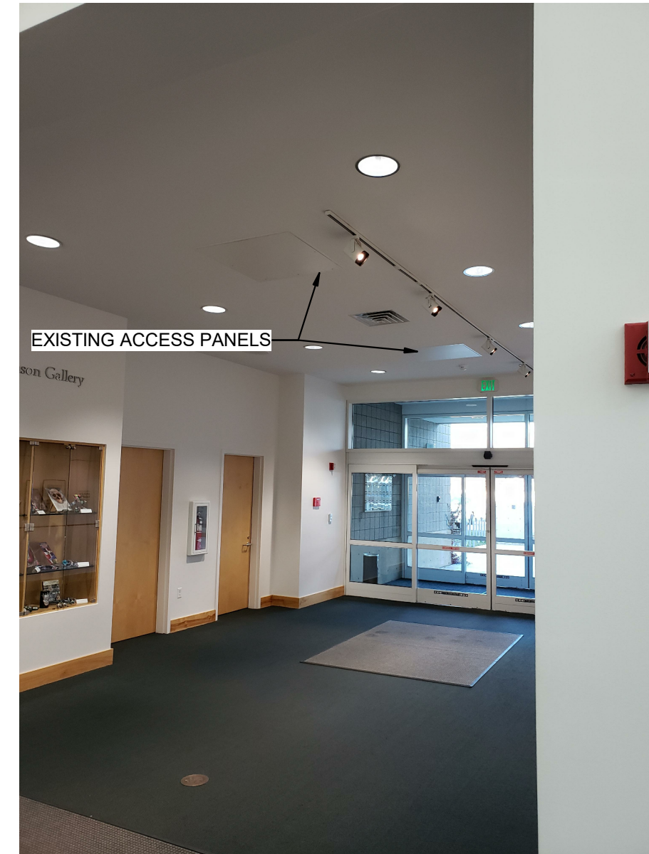
4 PHOTO 3 - EXISTING LOBBY SCALE: 1/8" = 1'-0"
