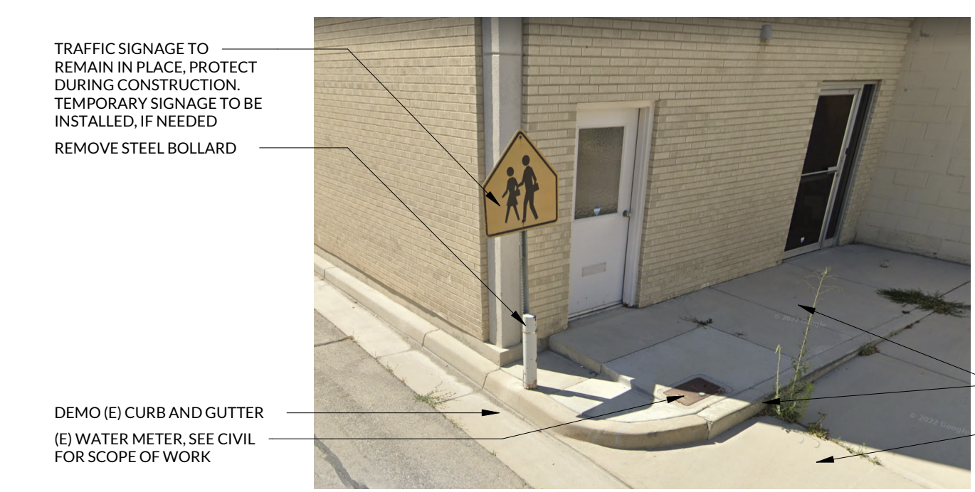
02 (E) EXTERIOR CONDITIONS - PHOTO NTS
