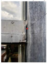
Remove existing all—silicone sealant and provide new silicone sealant. Clean all exterior windows frames and glazing.
