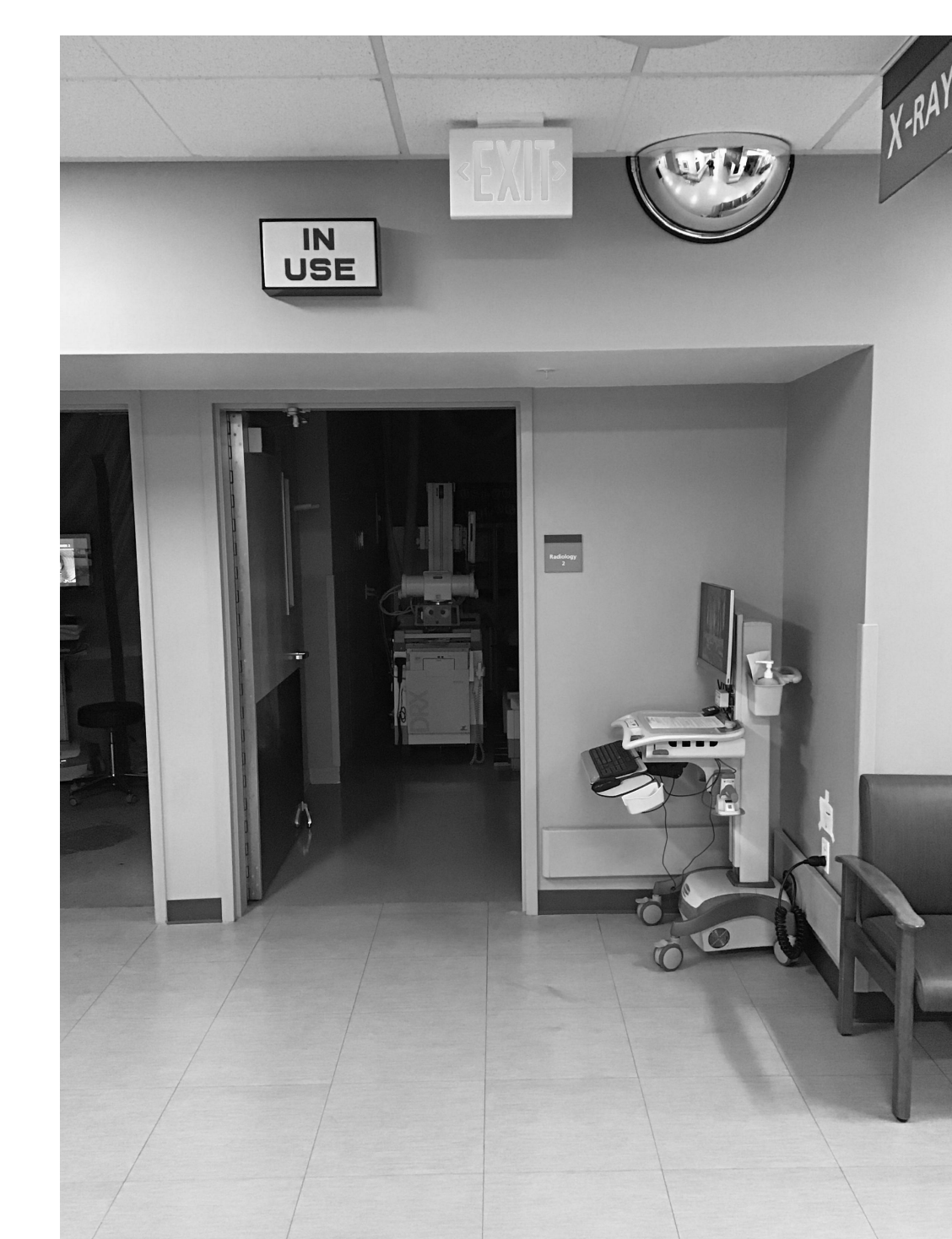
X-RAY ROOM ENTRANCE (Existing signage to remain)
