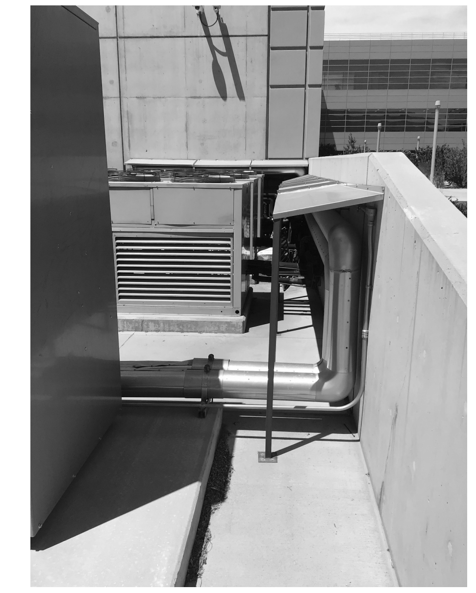
EXISTING METAL COVER STRUCTURE
