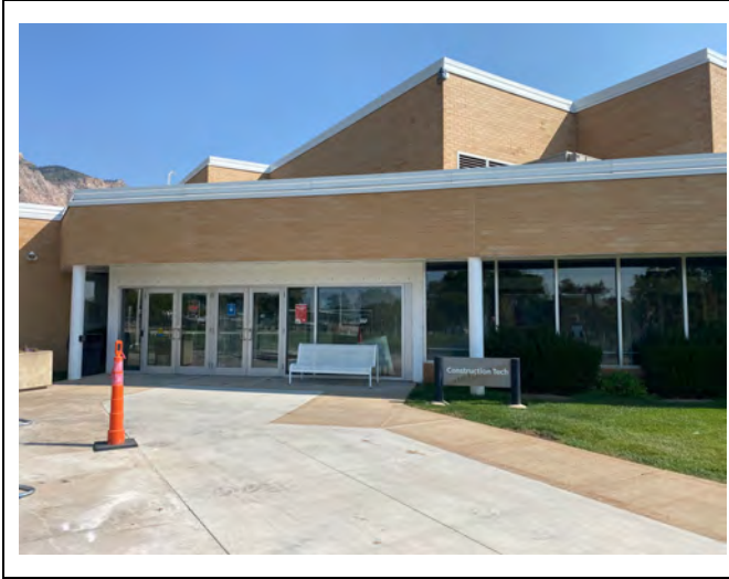
PHOTO 1: Ogden-Weber Technical College Construction Technology Building
