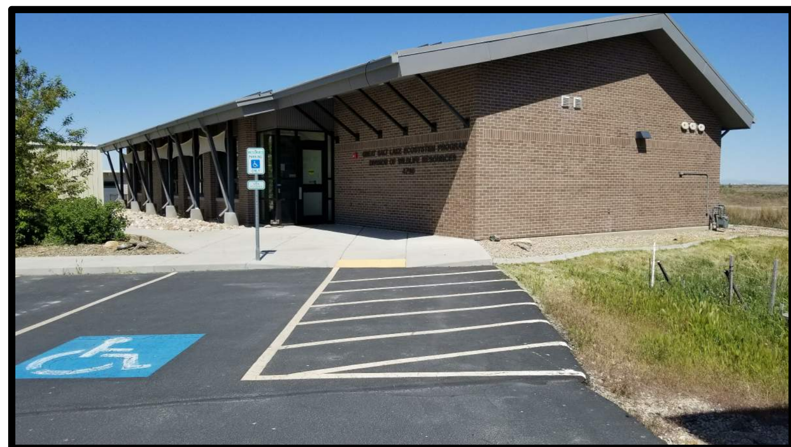
SOUTH-EAST CORNER OF EXISTING BUILDING
