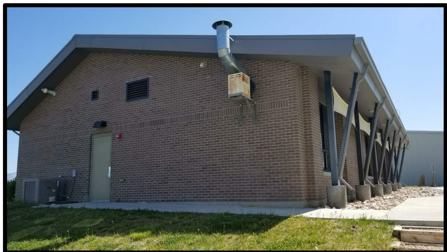
SOUTH-WEST CORNER OF EXISTING BUILDING
