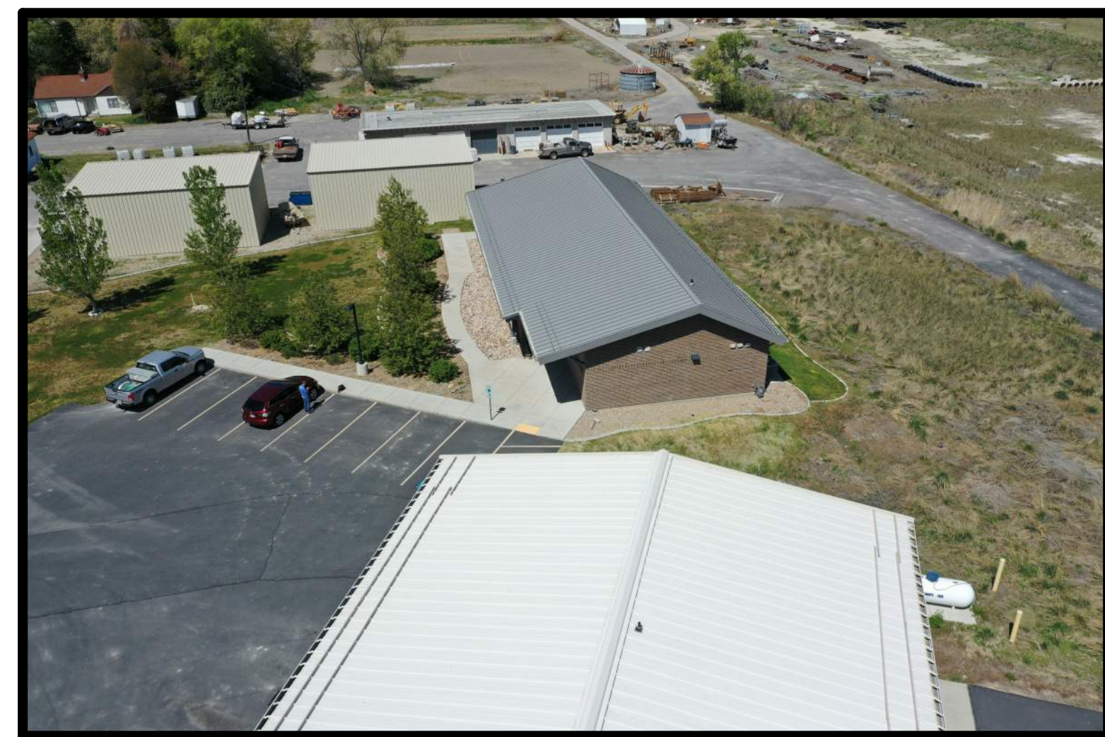
AERIAL VIEW - EAST SIDE OF EXISTING BUILDING
