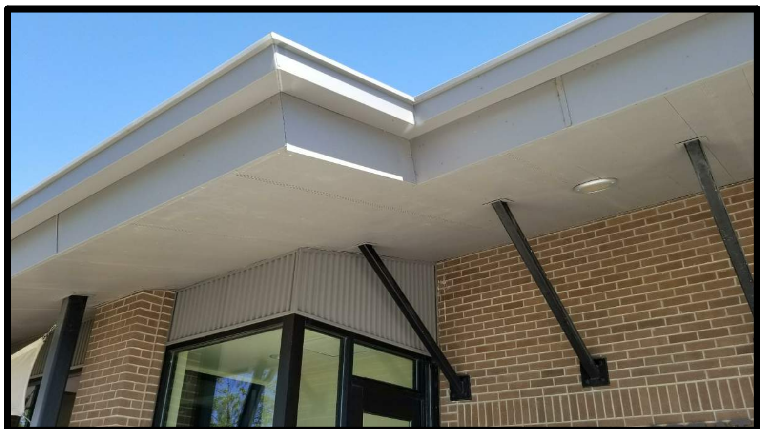
SOFFIT CONDITION AT THE MAIN ENTRANCE TO THE EXISTING BUILDING
