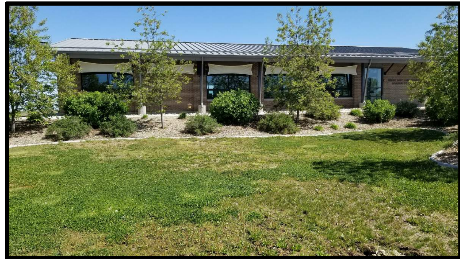
SOUTH SIDE OF THE EXISTING BUILDING
