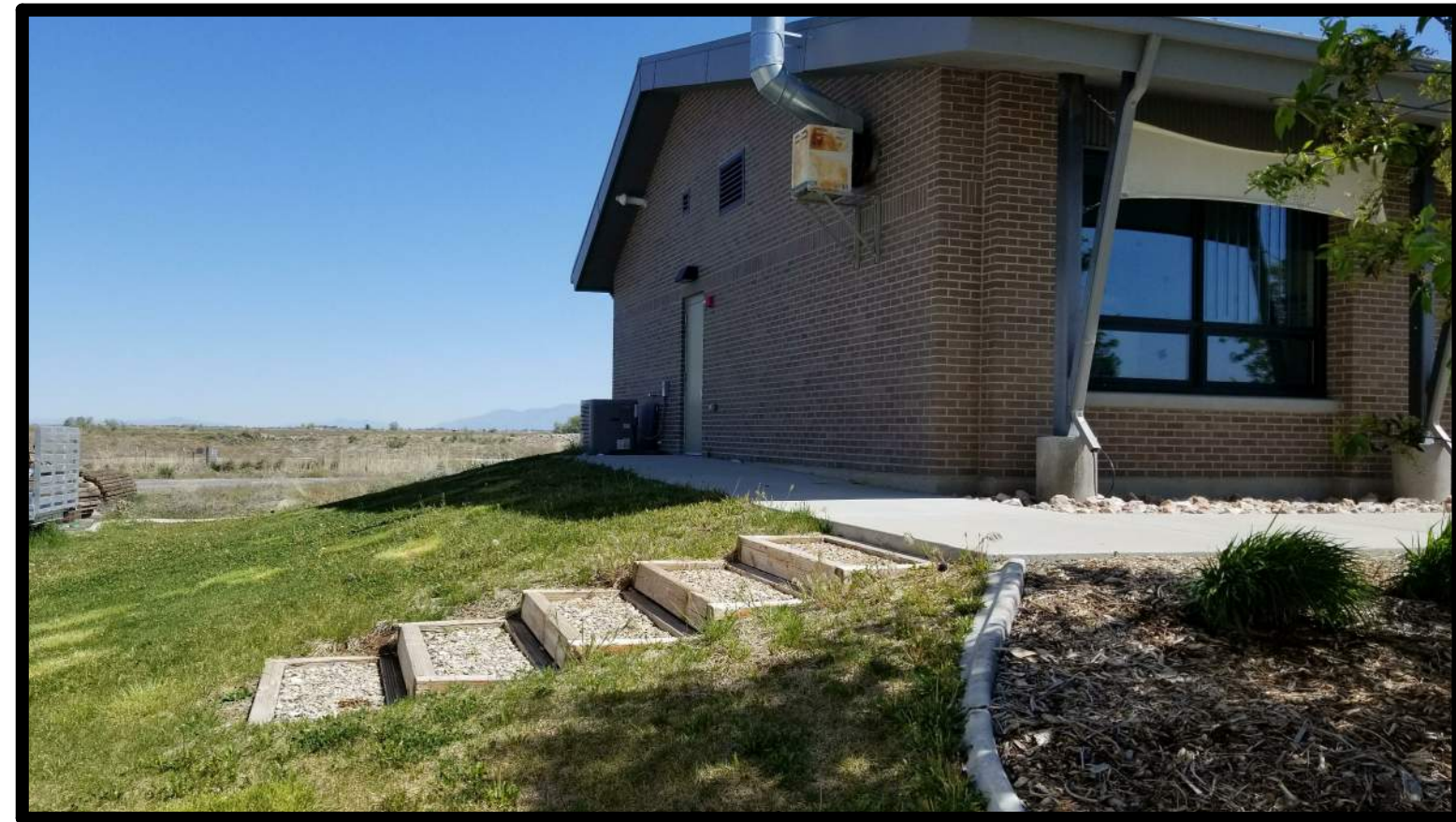
SOUTH-WEST CORNER OF EXISTING BUILDING
