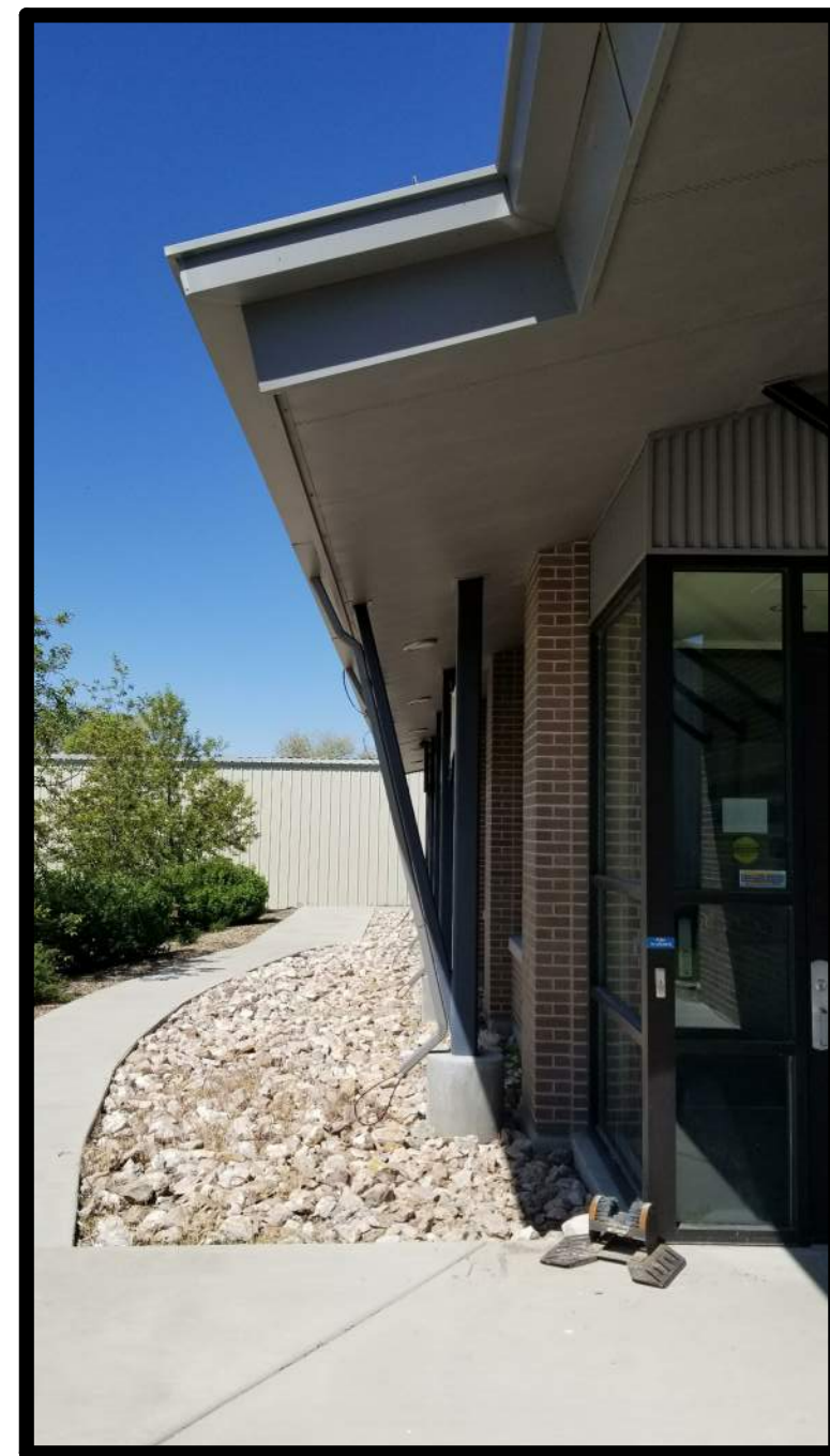
VIEW LOOKING DOWN THE SOUTH FACE OF THE EXISTING BUILDING SHOWING THE EXISTING ROOF OVERHANG THAT IS TO BE CUT OFF
