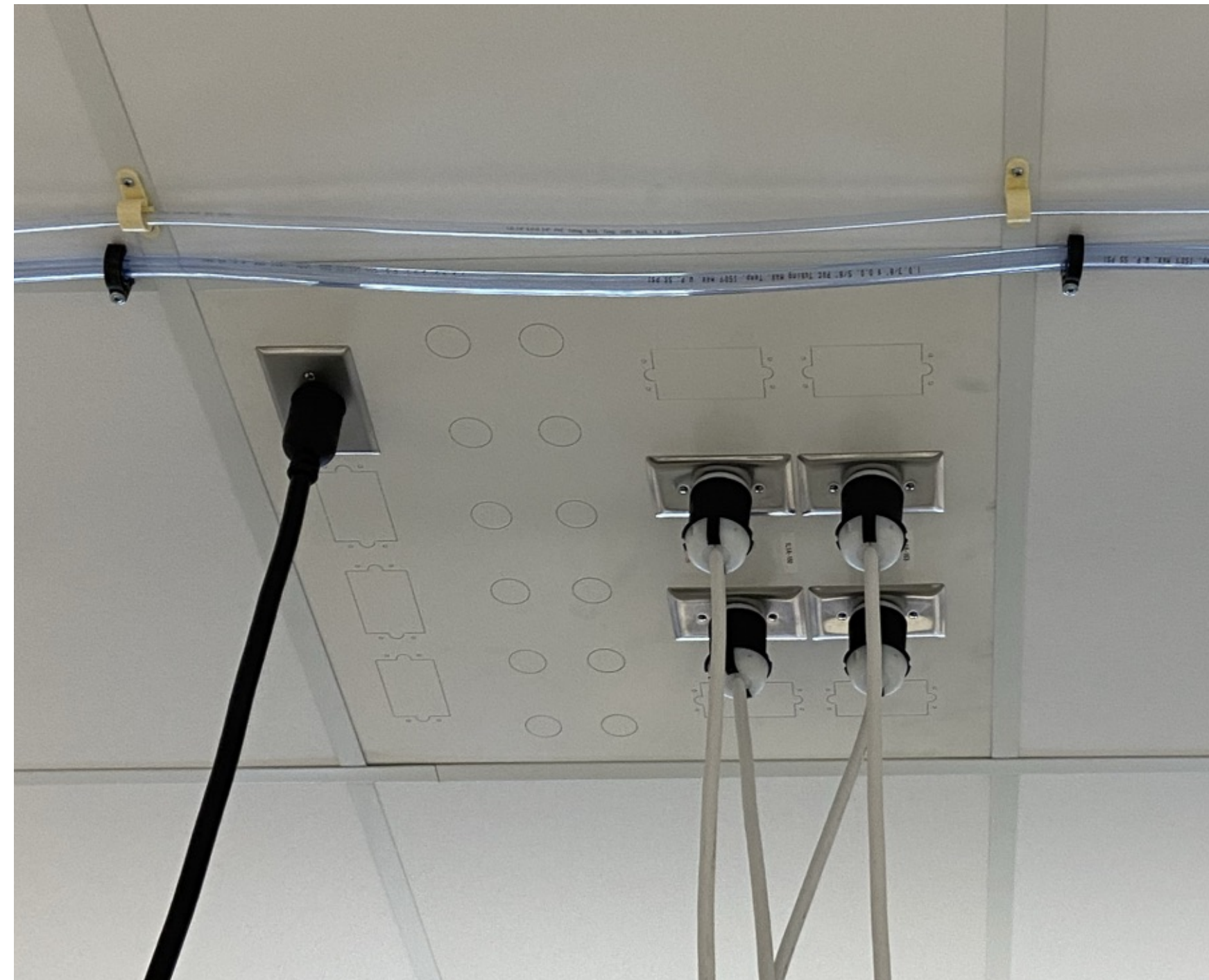
C2: EXISTING ELECTRICAL CEILING PANEL
