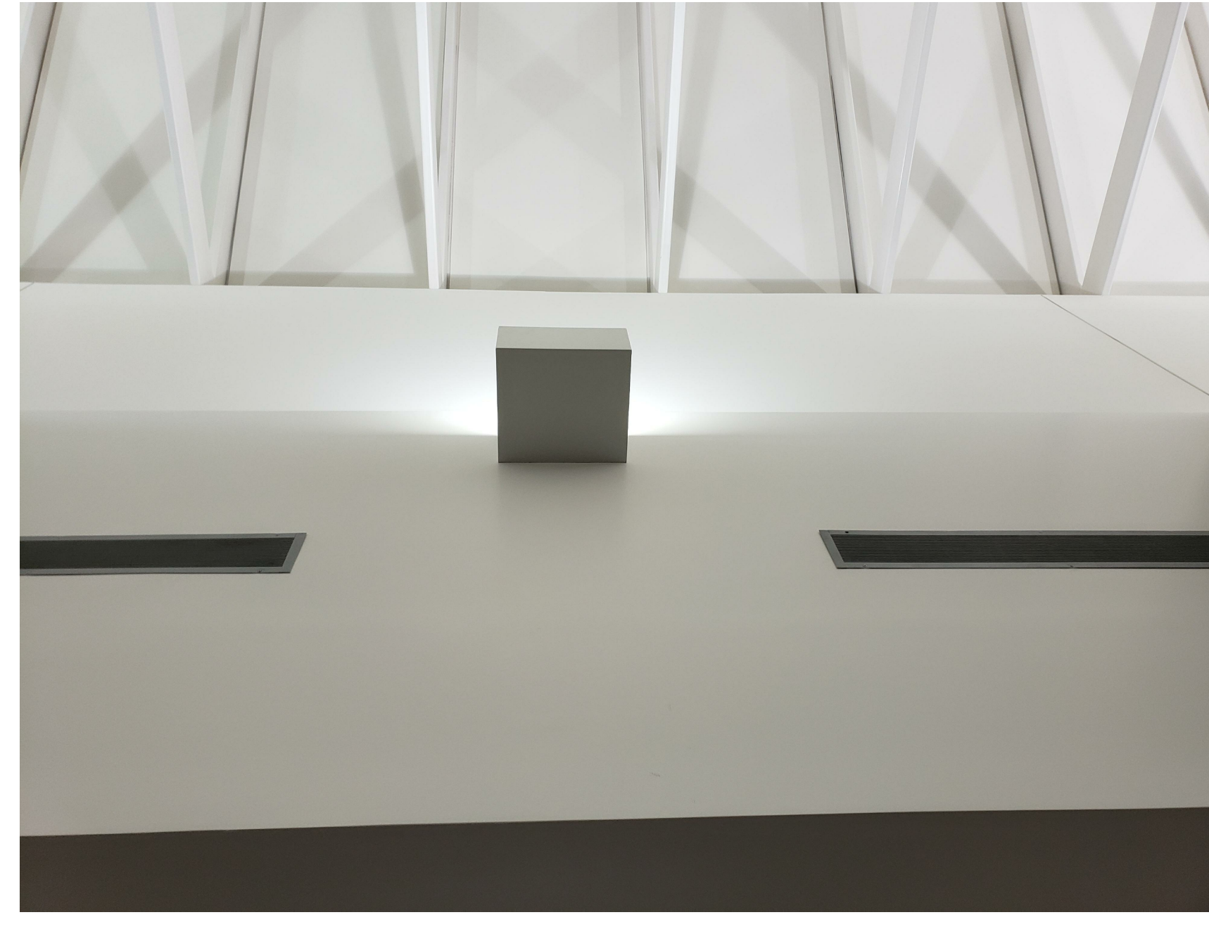
3 PHOTO3 - EXISTING UPLIGHT SCALE: NTS
