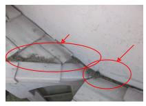
3.4 - The roof flashings/ flue pipes need to be sealed or serviced. They are comprised of metal that seals valleys and vents and other roof penetrations, and are the most common point of leaks. This is particularly true of the flashings on a layered roof, which are covered by the roofing material and which are even more susceptible to leaks.
