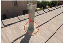
3.5 - The master bathroom exhaust vent pipe T-Top is absent and should be installed to prevent moisture intrusion.
