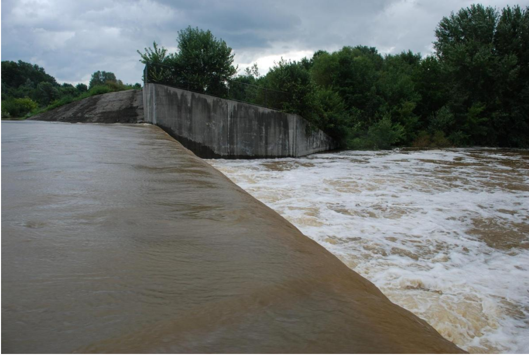
Looking from the top of the dam at the spillway during flooding conditions.
