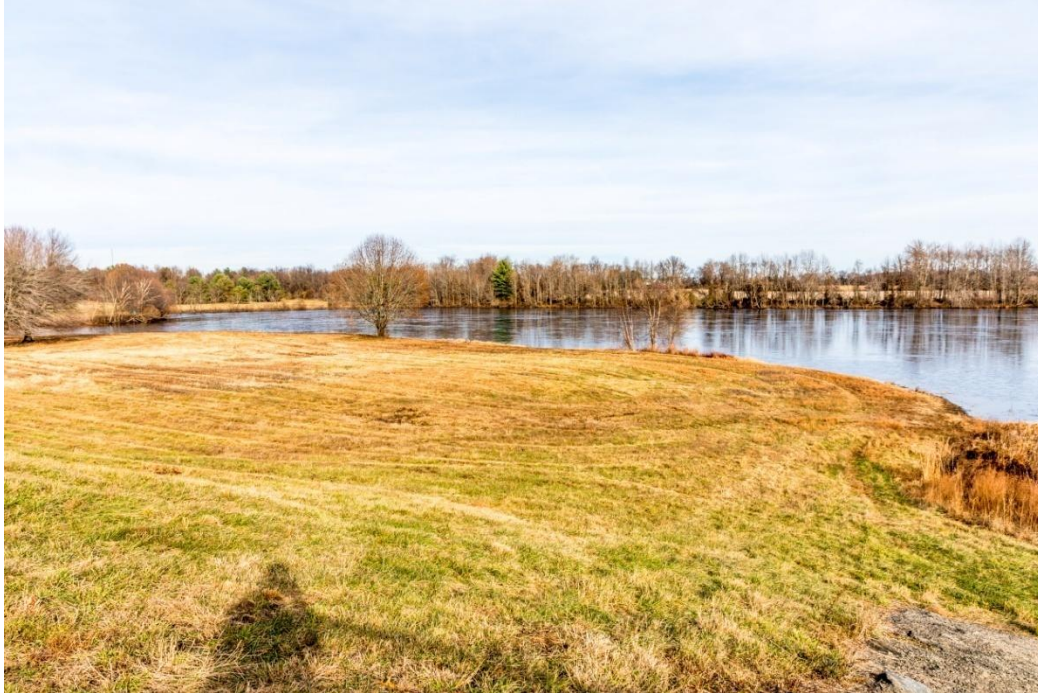
Looking from the top of the earthen dam standing next to the concrete dam
