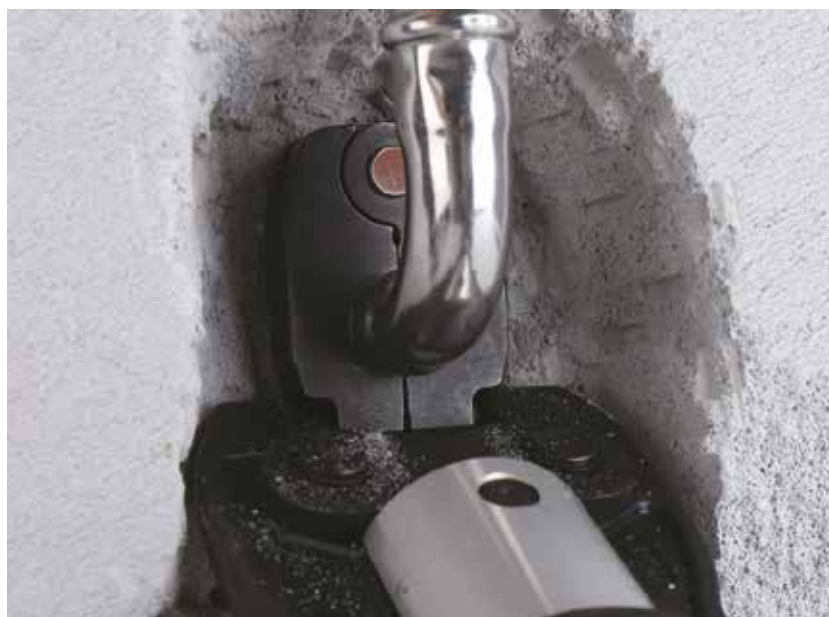
Spherical surface connection Swiveling 180-degree-flexibility
