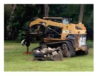
This very interesting machine was used to dig the post holes for the fence. United Fence let the poles set (dry) overnight before installing the wire.
