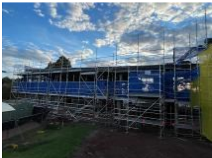
Progress on the new upper primary building
