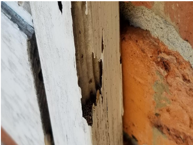
Drywood damage front shutter
