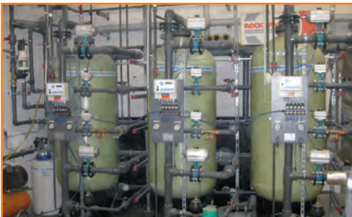
De-ironisation system for well water supply Dairy Berlin, Germany
