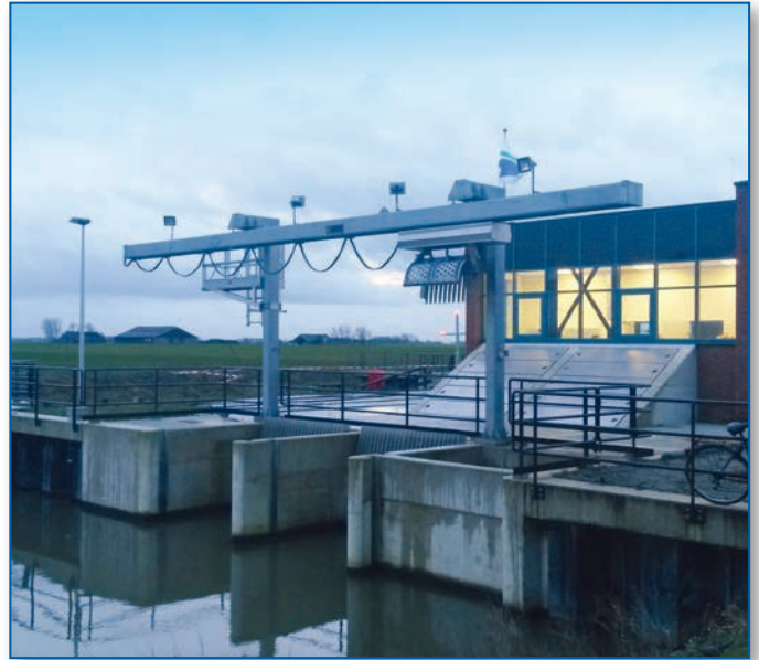
Dutch polder drainage station
