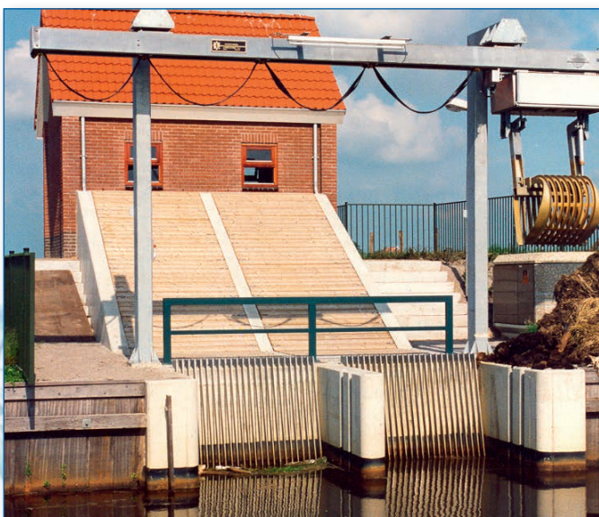
Polder drainage station Venhuizen, The Netherlands
