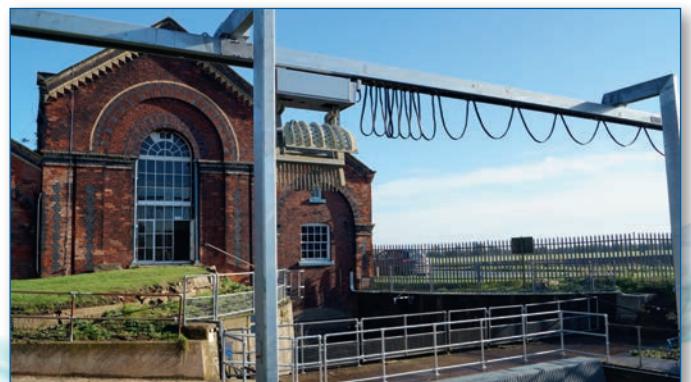
Pumping station with LANDY screen cleaning equipment
