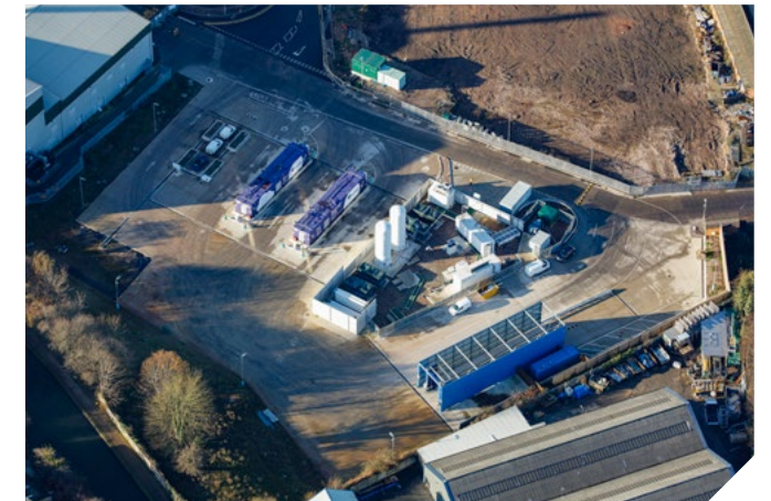
Image courtesy of Tyseley Energy Park
