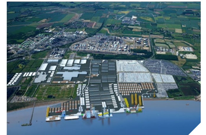
Image courtesy of Able UK
