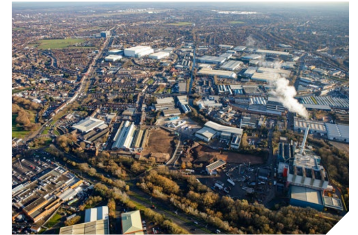
Birmingham East Corridor, Tyseley Energy Park
