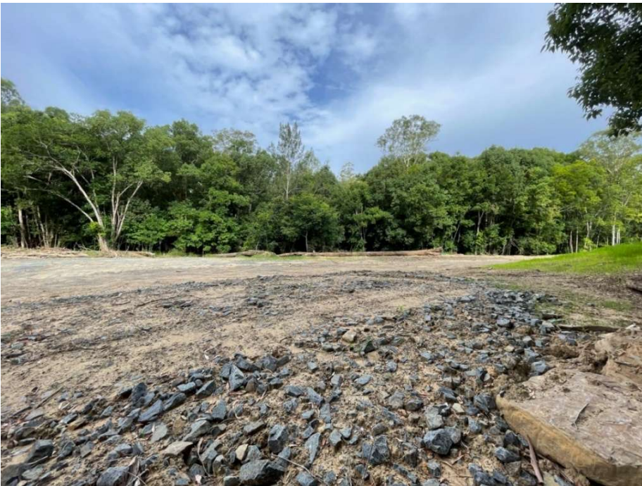
Below: early 2023. Bulldozed area along Opossum Creek.
