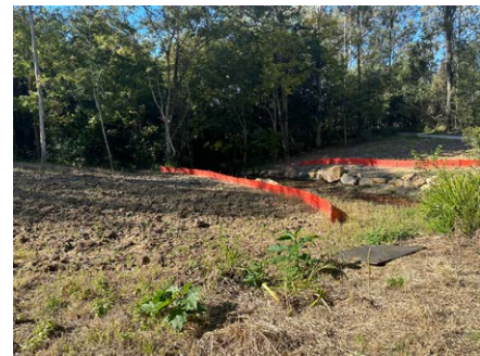
Weed treatment and apply gypsum to soil surface prior to mulching.
