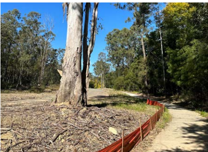
Install 4m wide mulched band tapered to 2m planted with Lomandra at 500mm spacings from large blue gum to start of rock wall.
