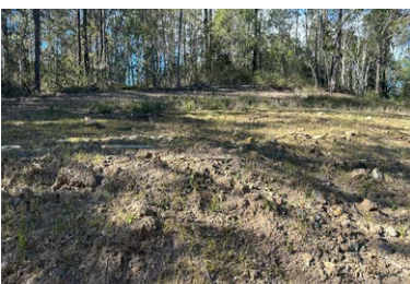
Access track requires rock removal, blading and water diversions installed.
