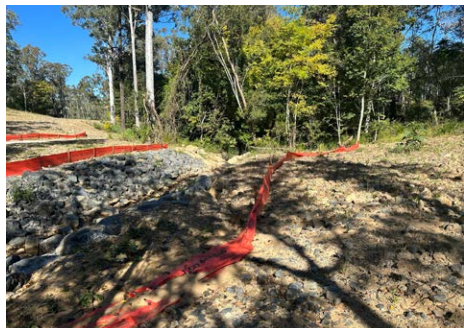
Reinstate sediment fence to functionality.
