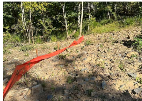
Reinstate sediment fence to functionality.
