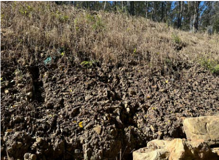
Repair eroded rills along the batter.
