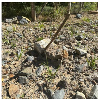
Metal objects such as reinforcing steel to be removed from site.
