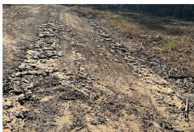
Access track requires rock removal, blading and water diversions installed.
