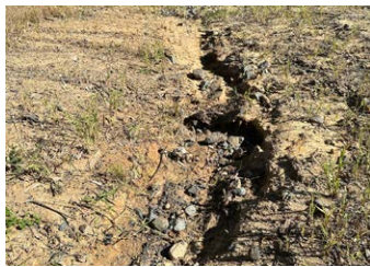
Install rock check drains into eroded rills.
