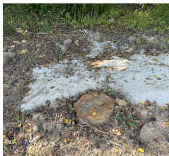
Excess concrete slurry to be removed from site.
