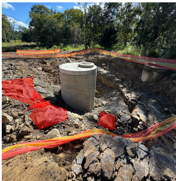
Phase 1 - Remove any large rocks and debris
