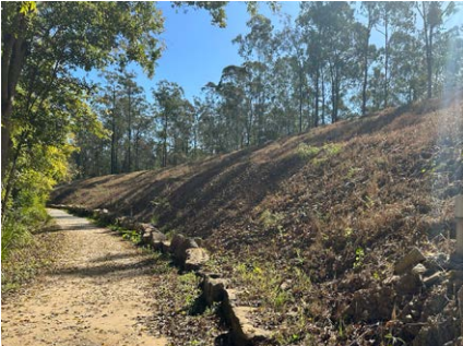
2m wide band of mulch to be installed and planted out with Lomandra hystrix.
