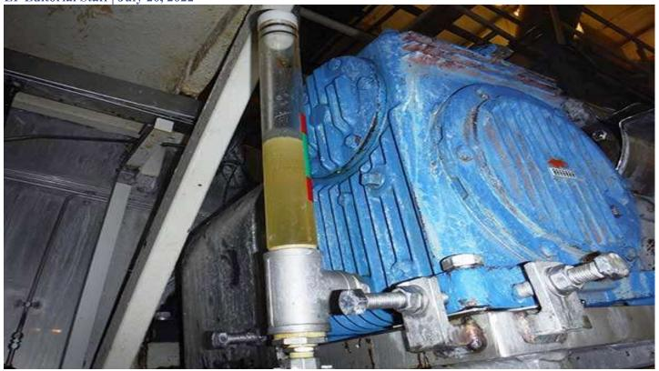
Entrained air, visible in this sight glass, can affect the bulk modulus of hydraulic fluids, which in turn affects their compressibility.
