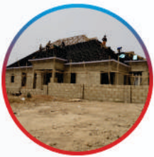
Roofing Services (Tilcor, Rain Gutter)
