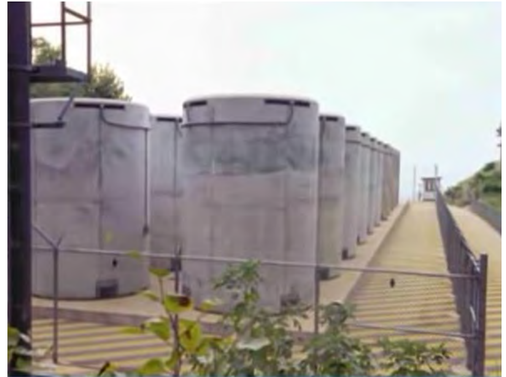
Dry cask storage for spent fuel at nuclear energy plants
