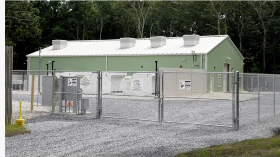
The 5-megawatt battery storage unit, located in East Hampton, has been out of service since a fire in May. Credit: Veronique Louis
