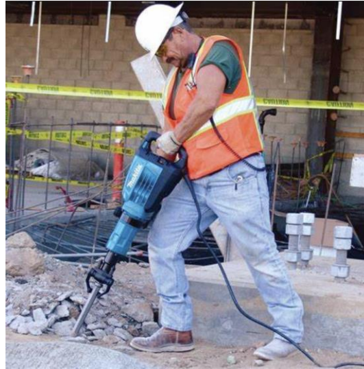
JACKHAMMER IS 102DB
