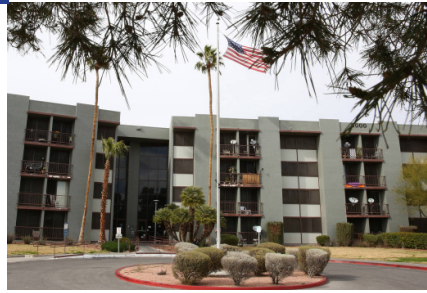
James Down Towers
