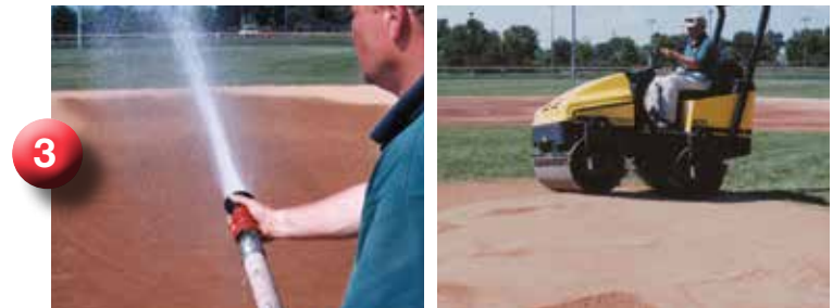
Moisten infield and roll with mechanical or hand roller.
