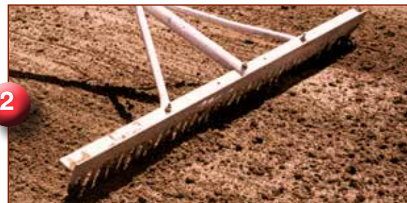
Step 2: Rake or drag to uniform layer over puddles and wet areas
