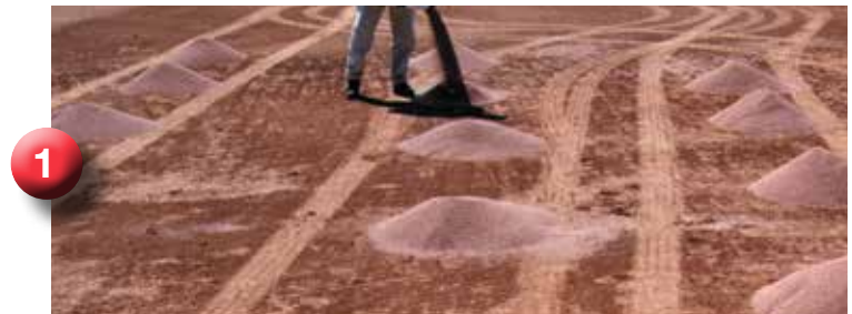
Position recommended number of bags on skinned area. Empty and spread with drag mat.
