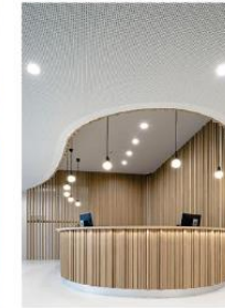
PERFORATED METAL CEILING WITH BLACK TRIM RECESSED LIGHTING
