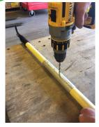
Use a  $\frac{1}{4}$  inch drill bit to drill completely drill through the pole through the 4 holes in the sleeve.
