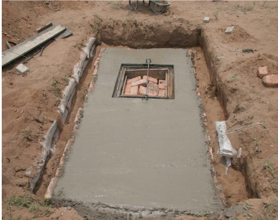
Figure 4.7 The Burial on Mapungubwe, showing the opening that was to become the manhole that would enable access for future research. Source: Johan Nel, 2007.
