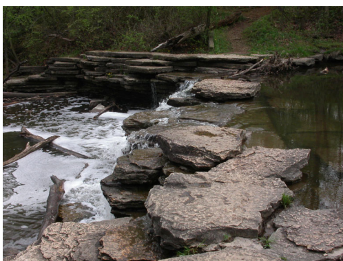
Two different views taken of the waterfall. All of the rock here was placed by man. You can tell by the large, flat, “stacked” appearance, with sharp edges on the thin sides, the rocks have no preferred orientation. If you took joint measurements the numbers would be random and trend every direction. Also quarrying marks such as blasting holes can be seen.
