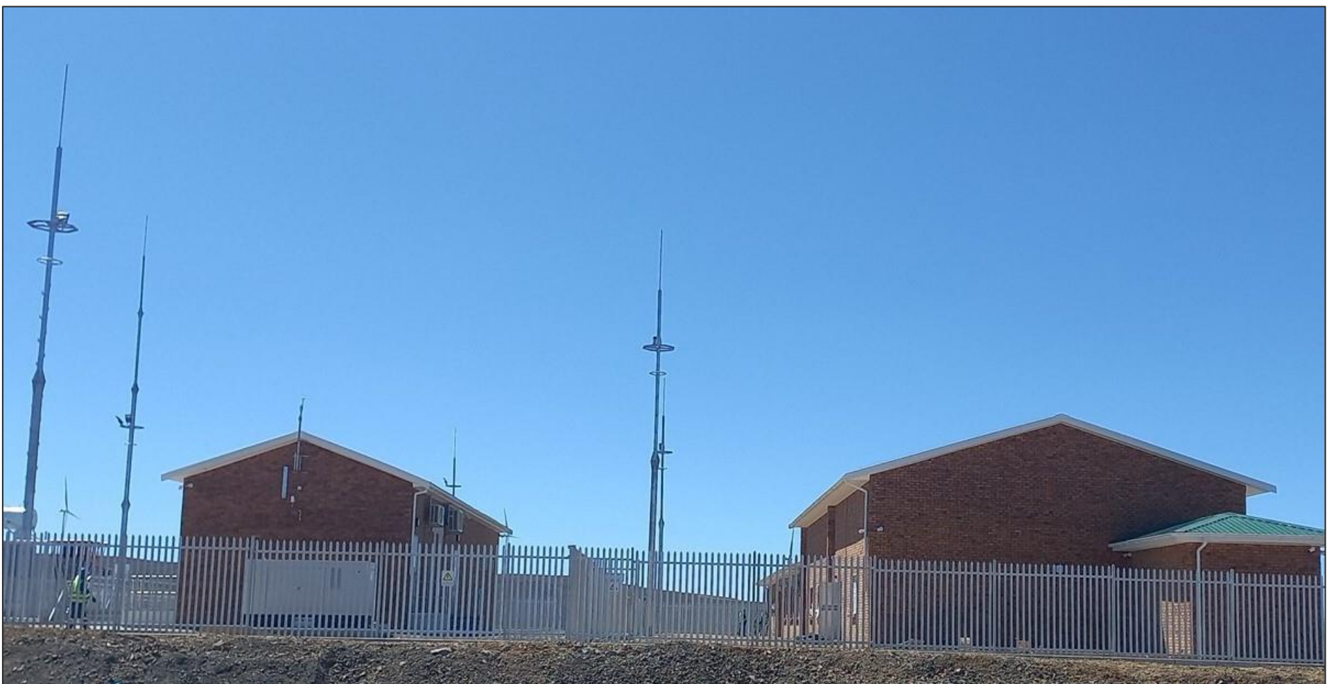
Figure 2: Completed Rietkloof Substation
