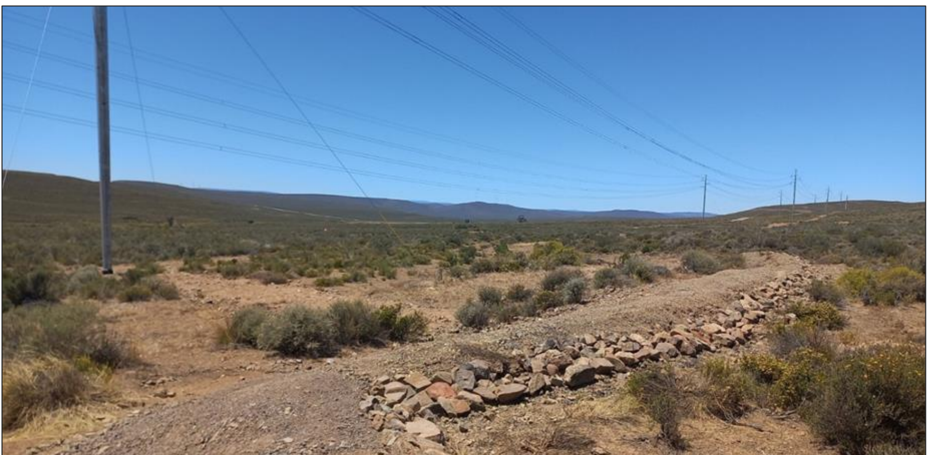
Figure 7: Stormwater diversion berm (photograph courtesy of Mahle Myaka)
