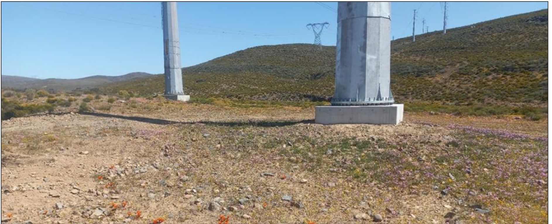
Figure 5: Rehabilitated Tower Foundation (photograph courtesy of Mahle Myaka)
