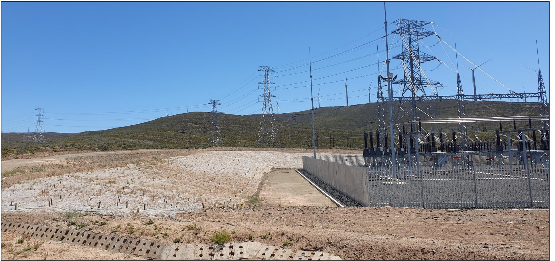
Figure 3: Rehabilitation at Bon Espirange Substation
