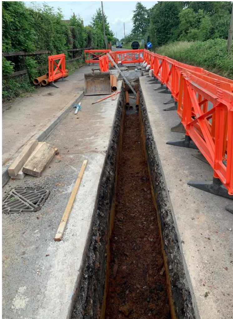
Drainage trench with TM
