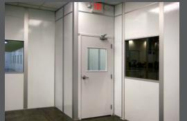
Temperature & contaminant controlling entrance,  $1^{3/4''}$ Light-Weight Aluminum System & FRP Faced Wall Panels
