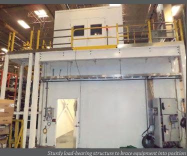
3" 16 gauge Heavy-Duty Steel System & 24 gauge painted Steel Wall Panels
