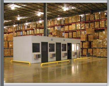
Four, warehouse management offices; constructed of InPlant's Standard Steel System & 3<sup>r</sup> Painted Gypsum Faced Wall Panels
