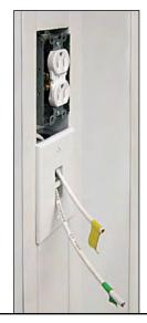
The Cover Plates in the Wiring Studs are cut to open sections for outlets and switches.
