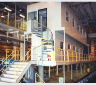
Two Story, 3" Heavy-Duty Steel System with Painted Steel Faced Wall Panels p to
