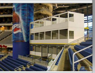
Partitioned suites on a mezzanine for media coverage; constructed of InPlant's Versatile Steel System & 13/4<sup>°°</sup> Painted Gypsum Wall Panels
