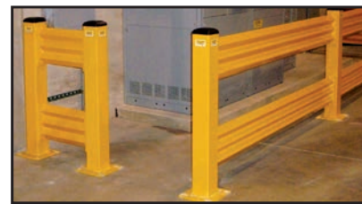
Guarding Electrical Panels
