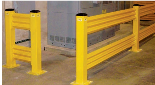
Guarding electrical panels
