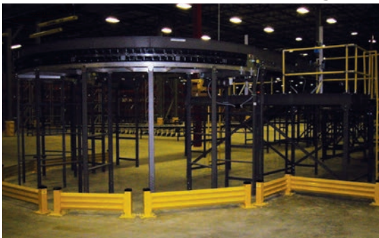
Guarding overhead conveyor
