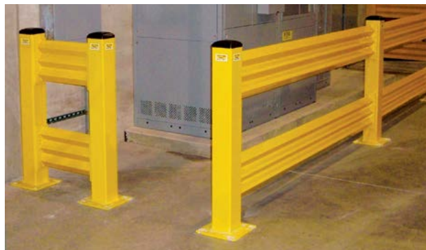
Guarding electrical panels
