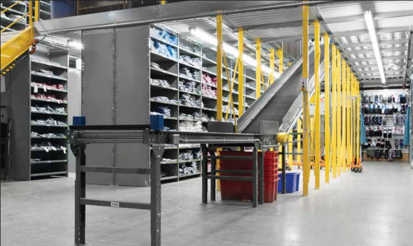
/ Integrated Conveyor in a Multi-tier System
