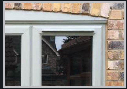
Trickle vent through a Rebated Sash
